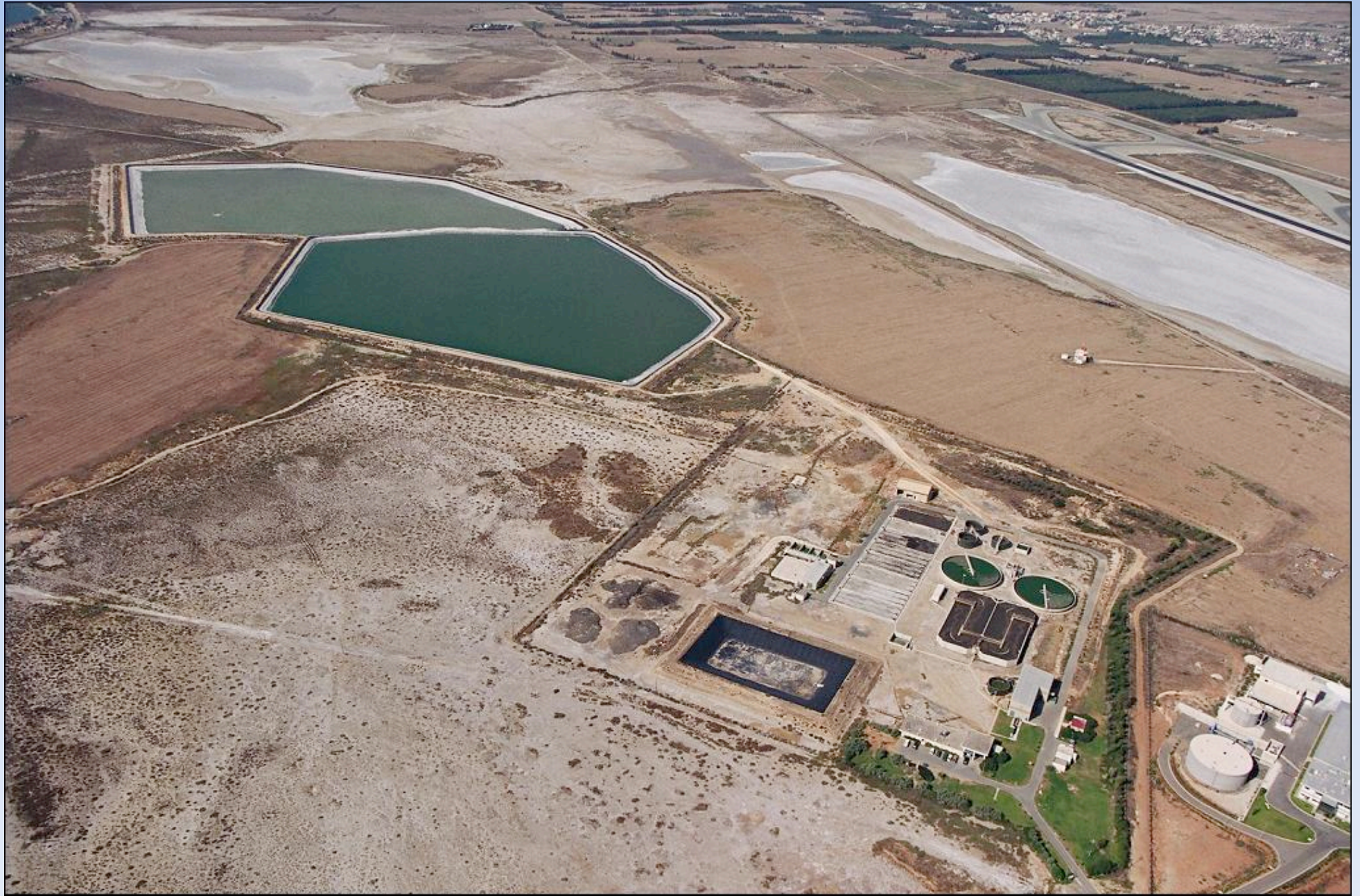
LARNACA WASTEWATER TREATMENT PLANT-SBL
