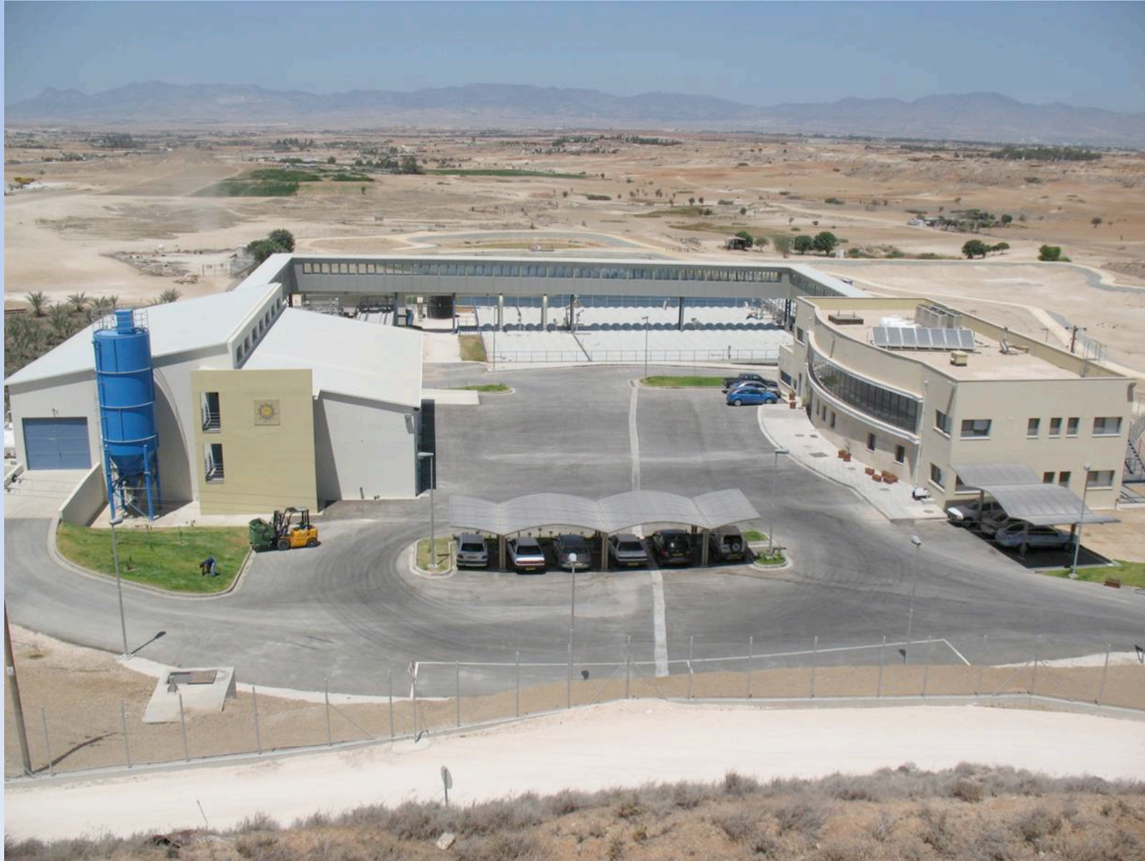
ANTHOUPOLIS WASTEWATER TREATMENT PLANT -SBN
