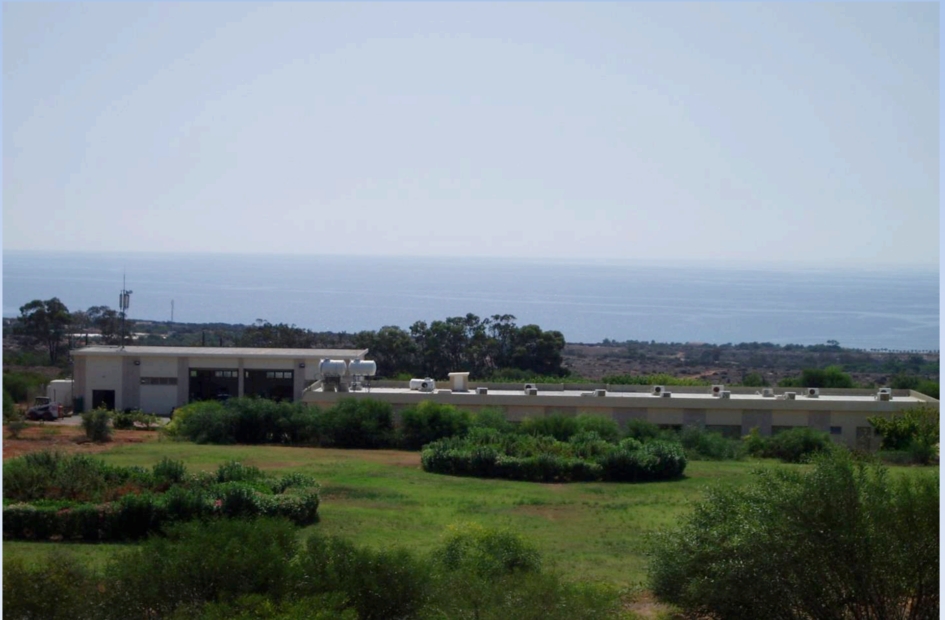
PARALIMNI-AYIA NAPA WASTEWATER TREATMENT PLANT
