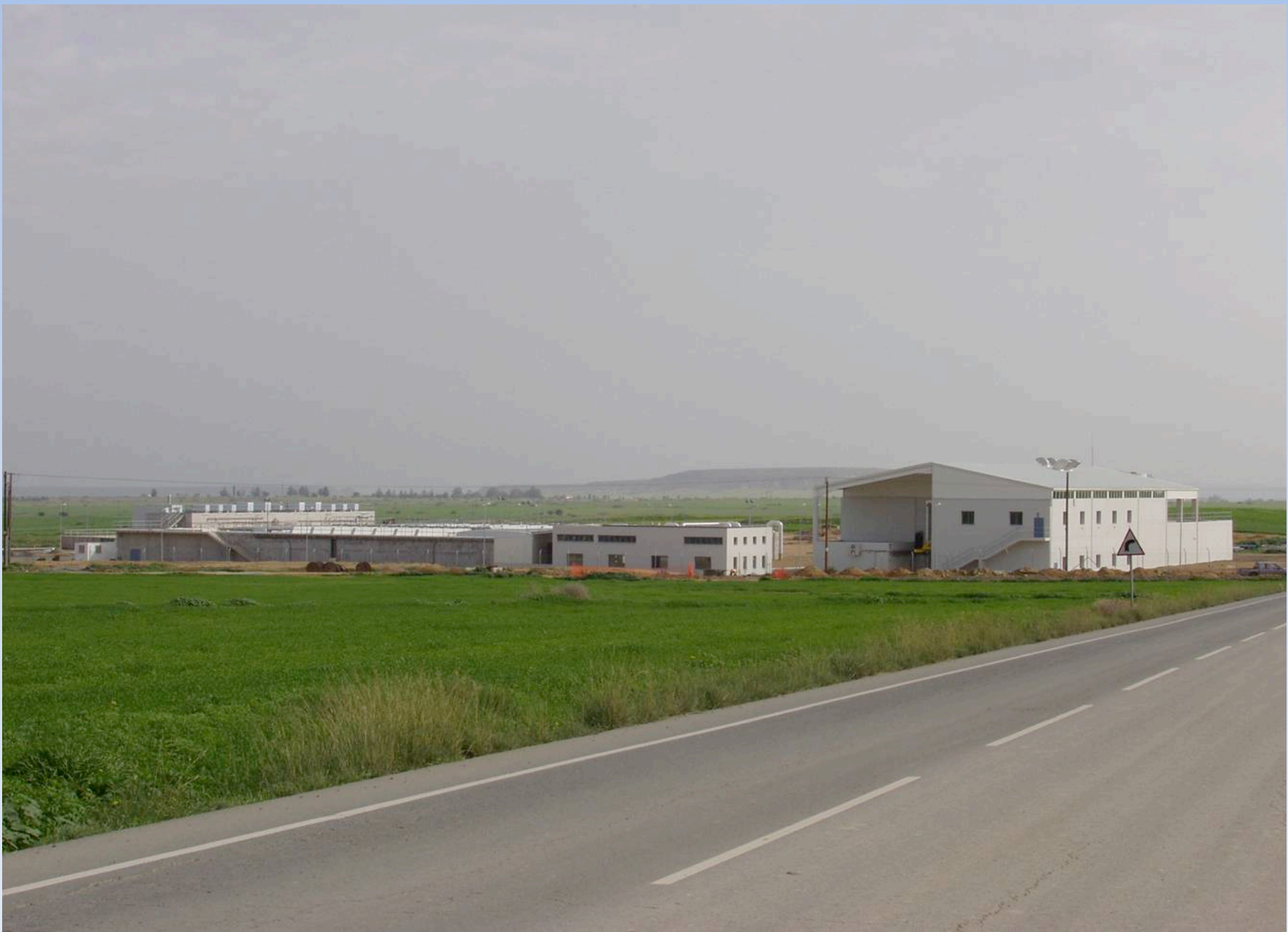
VATHIA GONIA WASTEWATER TREATMENT PLANT -SBN
